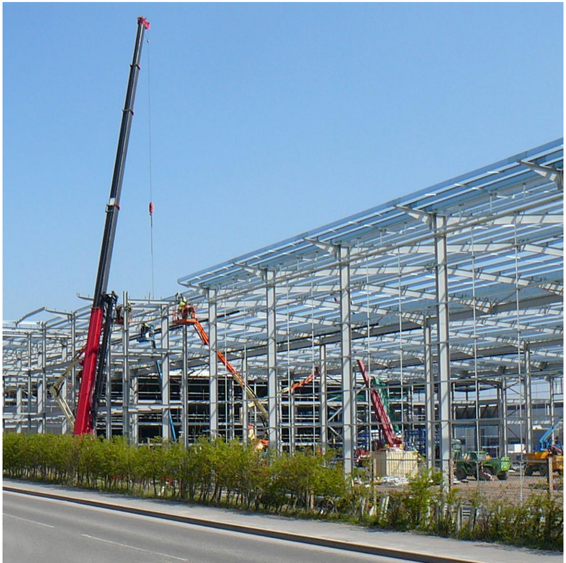
Photo 7: The Sports Direct distribution centre, under construction at Brook Park, Shirebrook
